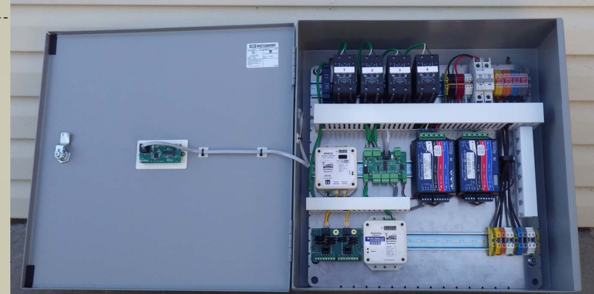
Right side (door): White piece is an LCD display for local viewing of status and diagnostics. Left side: Solid state relays and power distribution on top row. XRW2G sensor input module for meteorological and flow sensors, control board, and power / energy meters on middle row. And a RSTap internet gateway for remote monitoring on bottom row.
