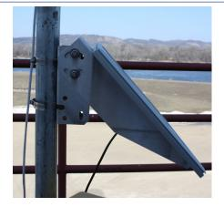
5. Insert bolt and flat washer from the inside out. Place a flat washer, lock washer, and hex nut on the outside. This orientation allows you to tighten the bolt with just one wrench.
