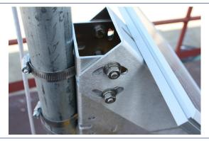
**6.** Adjust the tilt of the panel as desired, and tighten the bolts.
